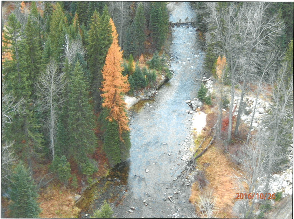
PHOTO #1 - VIEW OF CROSSING LOCATION-WOODS ON LEFT
